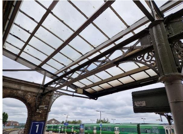
**Figure 5-9: Lattice Truss (nts)**
